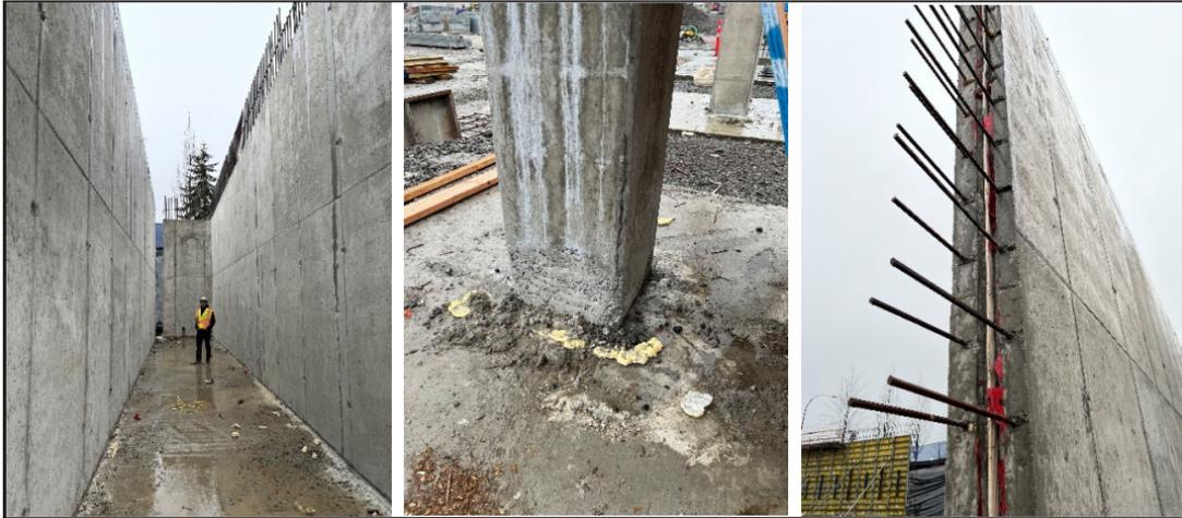
Concrete foundation retaining wall, column and wall segment
