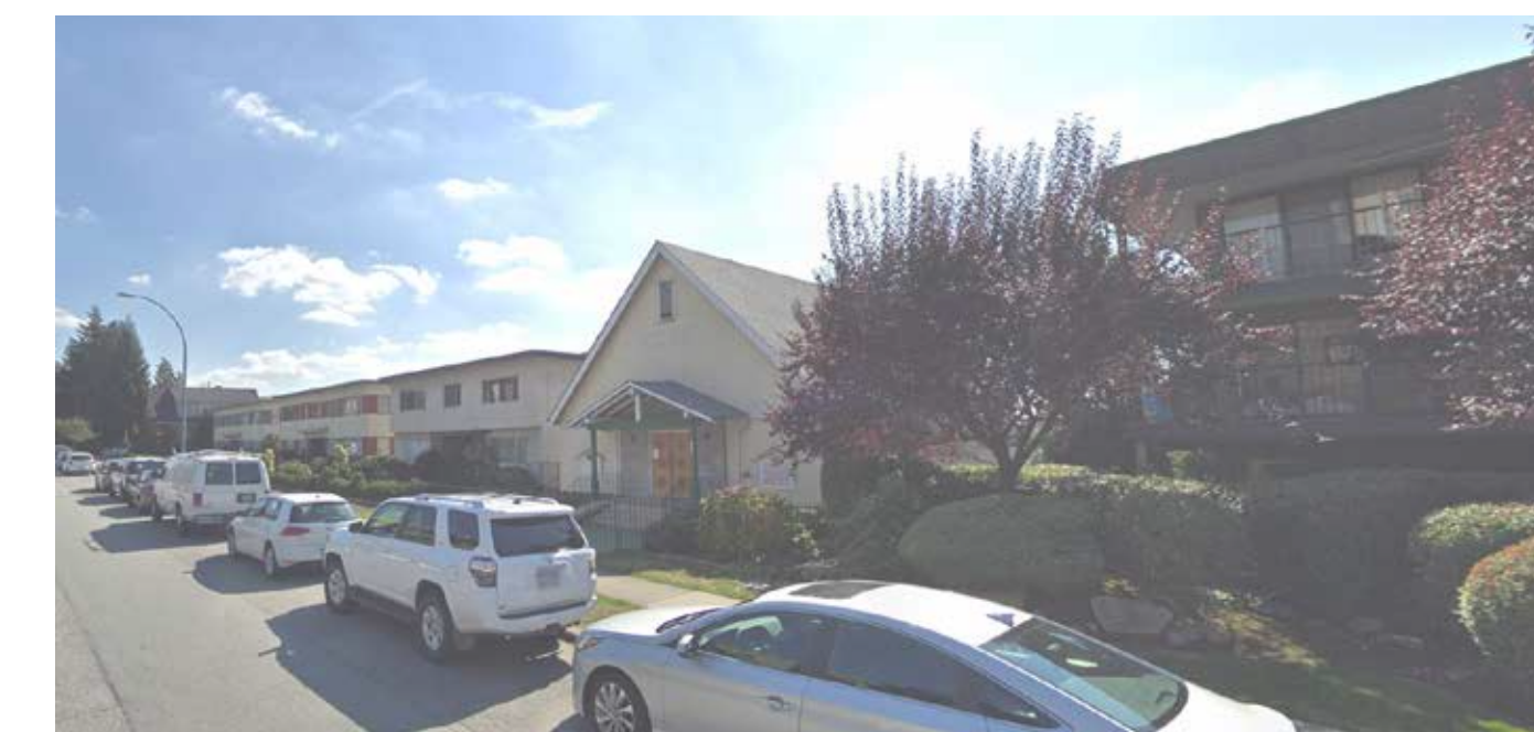
View Along E 4th St Looking East
