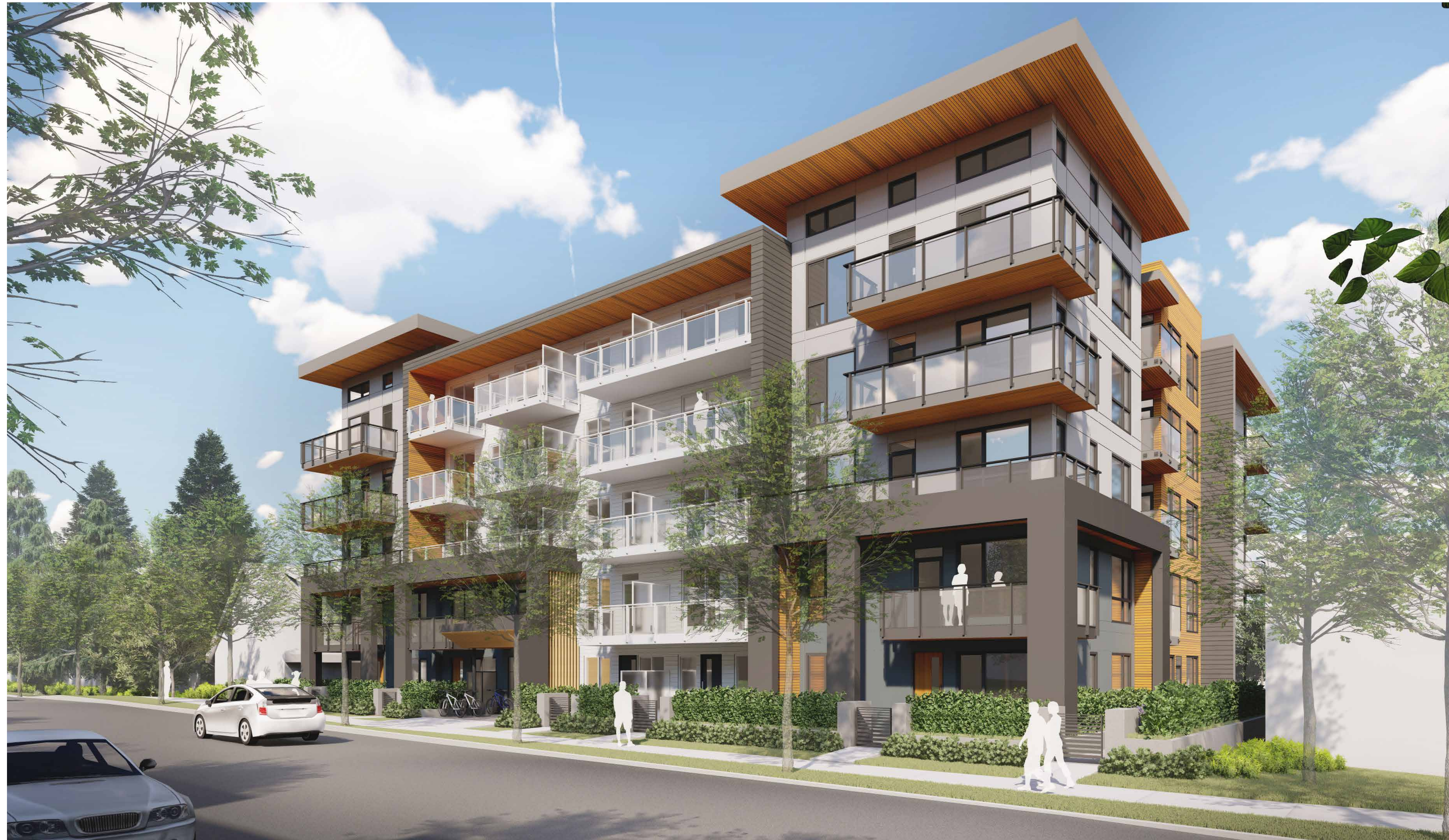
View from E4th looking South East at Front Entry
