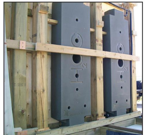
Example of above-ground rainwater tank: "HOG" tank
