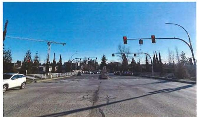
While it is possible to cross the highway on the sidewalk, the width of the sidewalk does not meet currently accepted design standards for pedestrian infrastructure adjacent to a high vehicle volume roadway. The sidewalk edges have low contrast against the roadway asphalt, making the safe pedestrian space difficult to discern by people with low vision. The letdowns at all access points north and south of the highway do not meet modern accessibility design standards.
