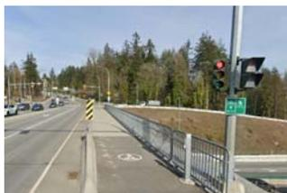
Revising existing bridge lane widths or configuration to accommodate protected active mode space (ex. Mountain Highway)
