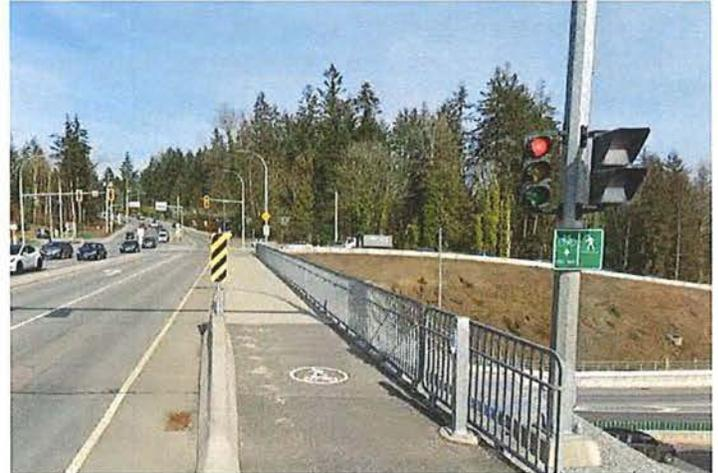
**Cantilevered Pathway:** Creation of a separate active mode facility connected to the existing interchange bridge.
