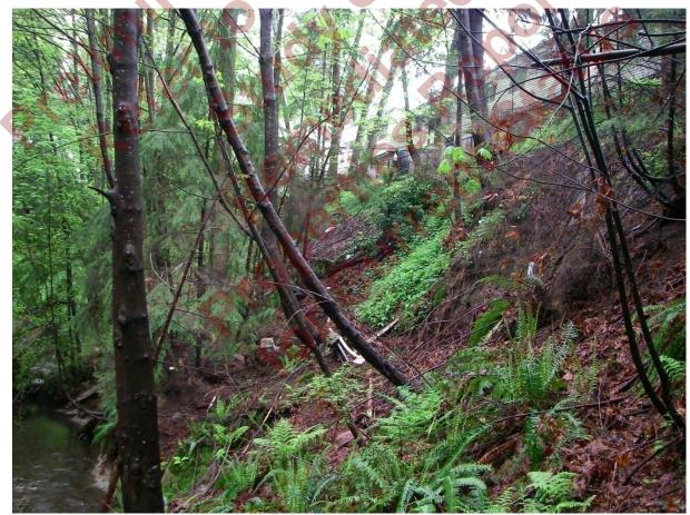
Photograph 7: Shallow earth sliding and stream erosion below Units 837-851, Westview Cres.
