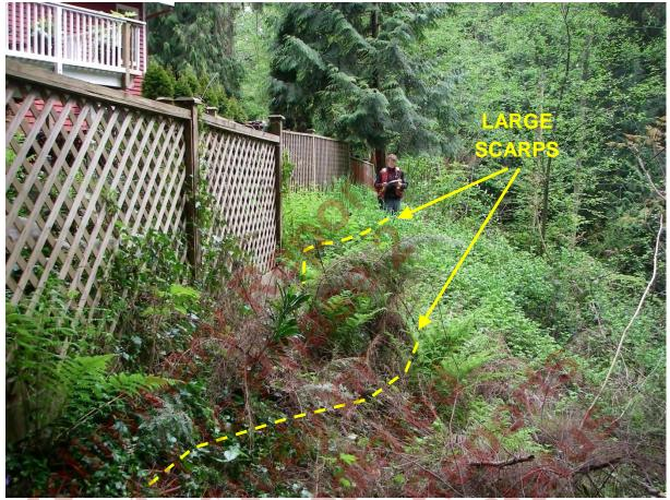
Photograph 8: View of Large Scarps along Crest of Slope, 1956 Wolfe St.
