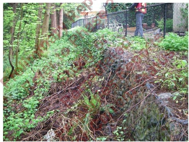
Photograph 6: Gabion wall at top of slope, 811-821 Westview Cres.
