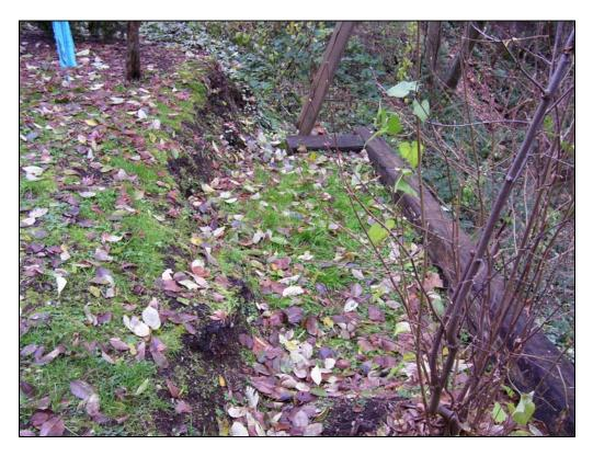
Plate 3: The separation behind the face of the retaining wall.
