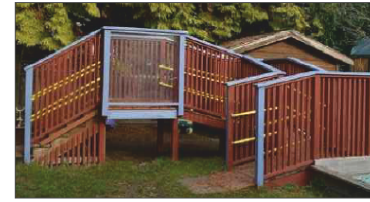
WOODEN RAMP AND STEP STRUCTURE, ALREADY BUILT, FLEXIGLASS ART SURFACE SCALE: NTS
