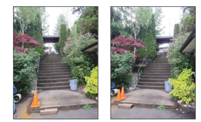
Photos of Existing Stair to East 3rd Street
