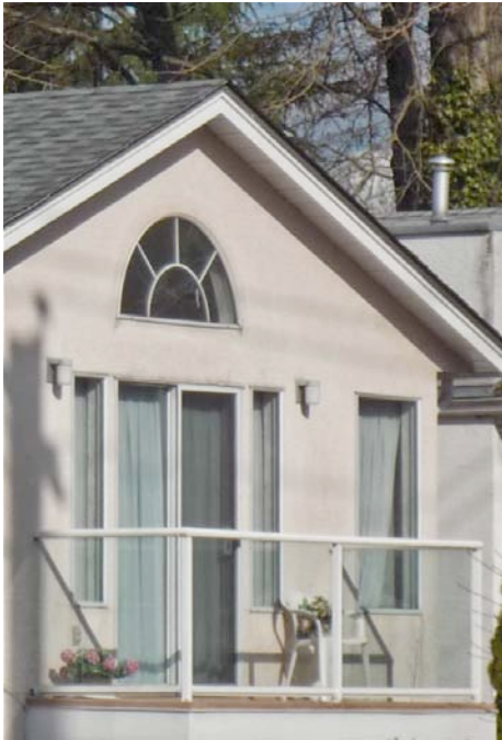
Inappropriate materials and window treatment
