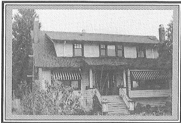
W. H. Parkins Residence 766 Grand Boulevard F. J. King, Designer 1930
