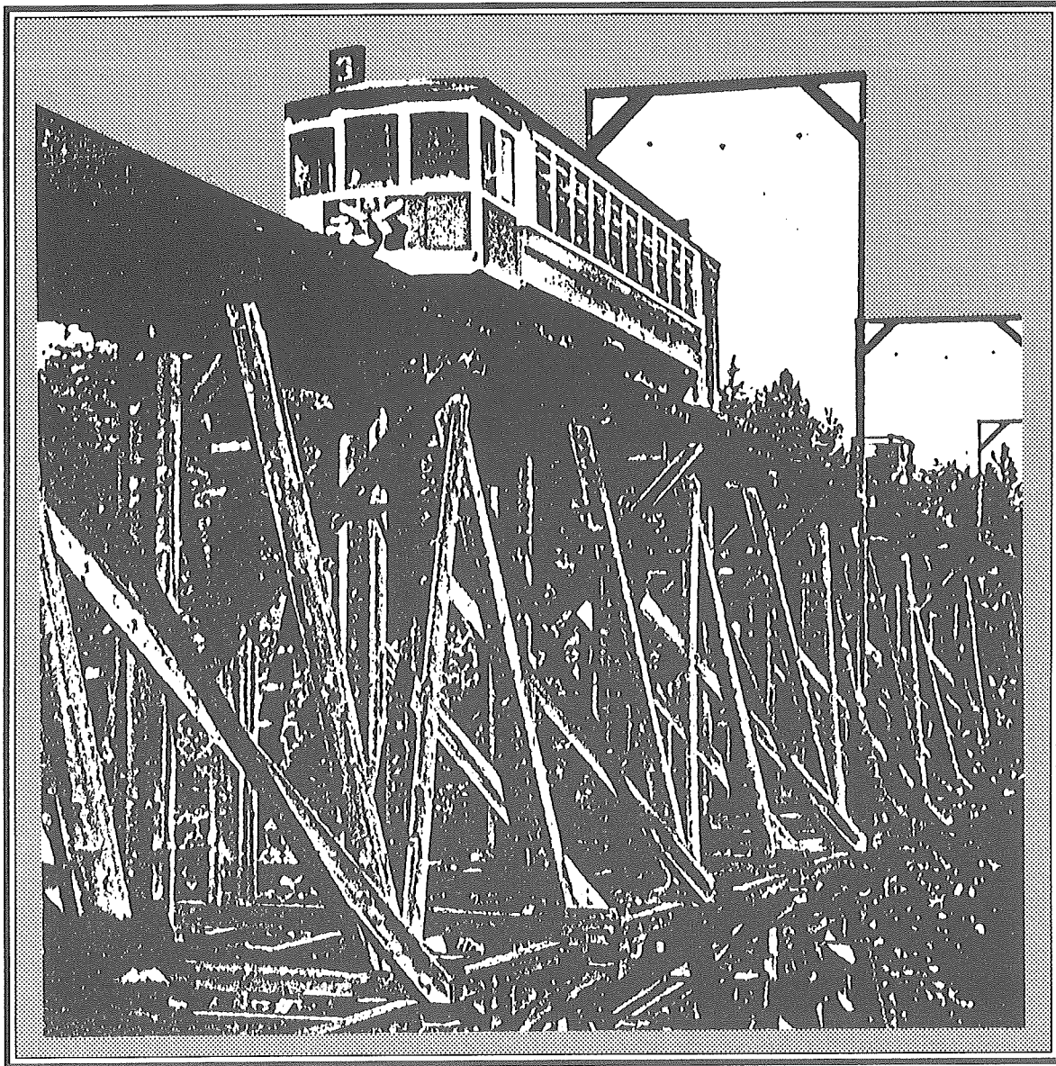
Above: The Mackay Creek Trestle. Source - North Vancouver Museum & Archives #6578
