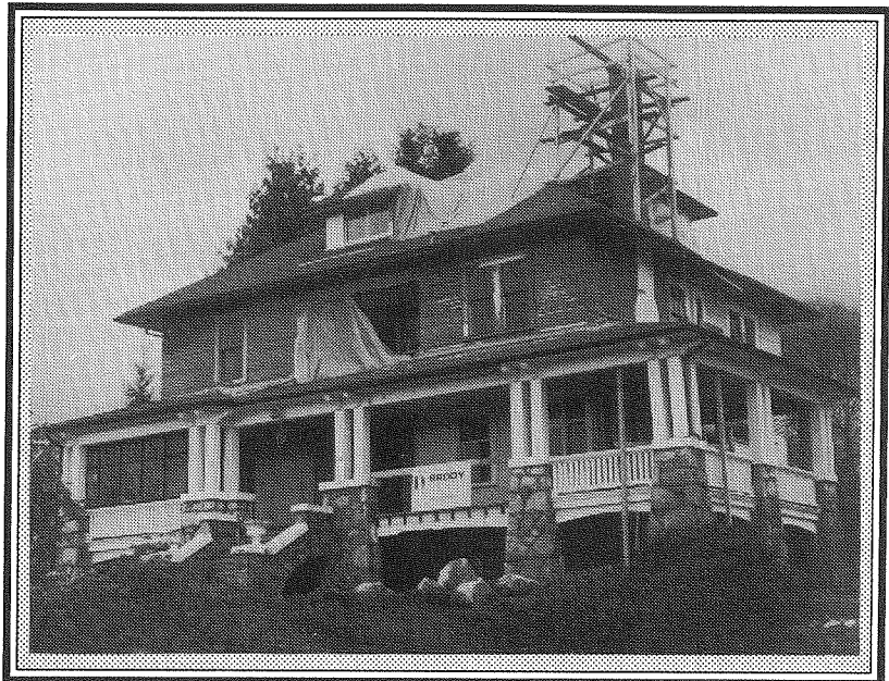
Above: The McNair Residence during restoration in 1994.
