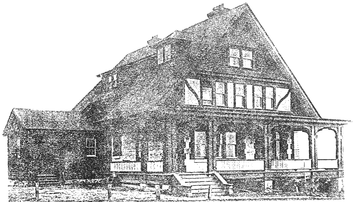
Above: The Hamersley Residence in 1906.
