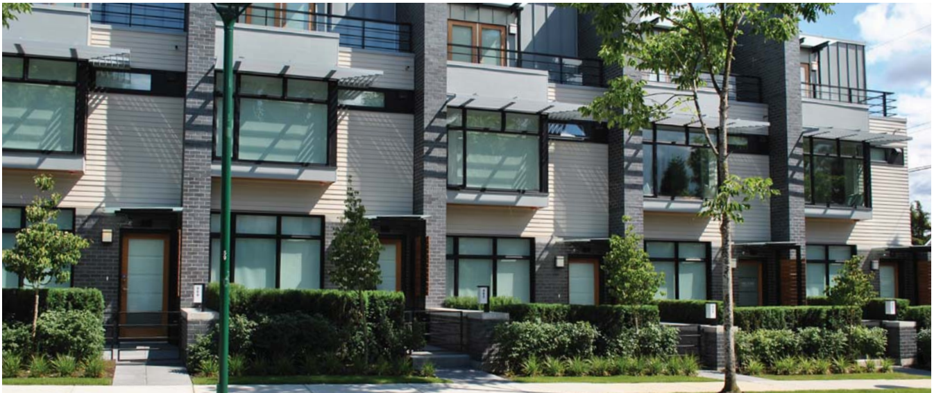
Figure 27 is provided to support the building envelope guidelines in this section. Detailed drawings of different building types are included in Part IV of the Moodyville Guidelines.
