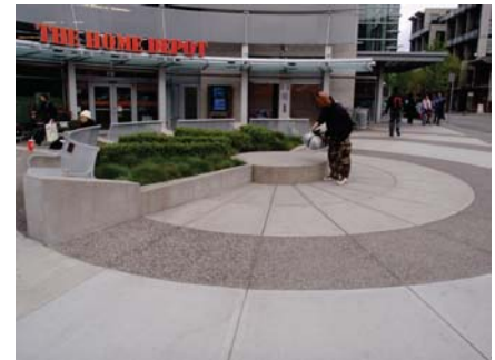
Corner treatment with exposed aggregate radial band
