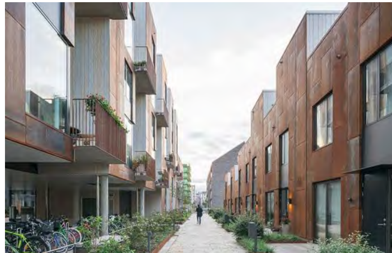
Zenhusen housing, Stockholm, Sweden
