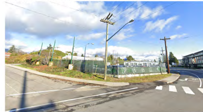
3. Building under construction
