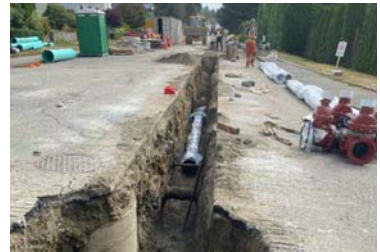
▲ West 27 th St. water main replacement [2024]
