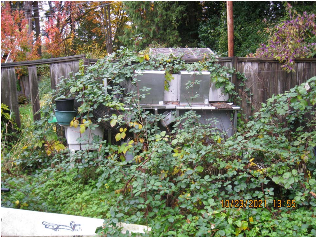
Rear yard, west side, looking west
