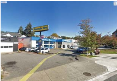
VIEW FROM MARINE DIRVE LOOKING EAST N.T.S
