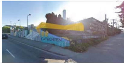
VIEW ALONG FORBES STREET LOOKING NORTH
