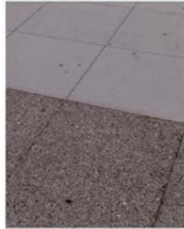
Broom Finish Concrete and Exposed Aggregate Concrete
