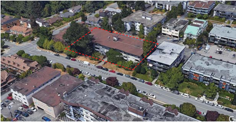
SUBJECT PROPERTY - OVERALL VIEW
