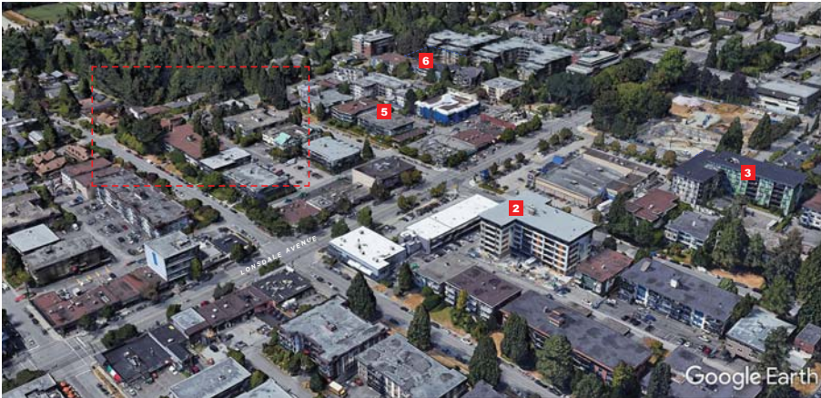
EXISTING SITE - AERIAL VIEW NORTH WEST
