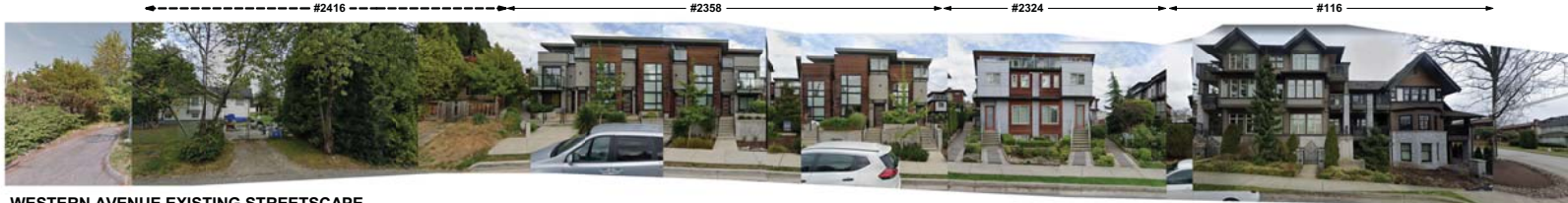
WESTERN AVENUE EXISTING STREETSCAPE
