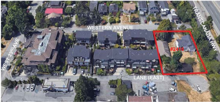
AERIAL VIEW - LOOKING WEST
