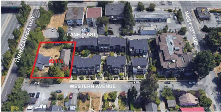
AERIAL VIEW - LOOKING EAST
