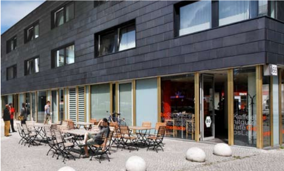
Expand on palette of materials through the use of highly sustainable and durable materials (fibre-cement panels, certified wood, high performance glazing).
