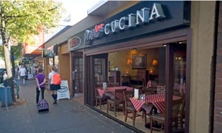
Design building facades to allow for flexibility in size and location of building openings.
