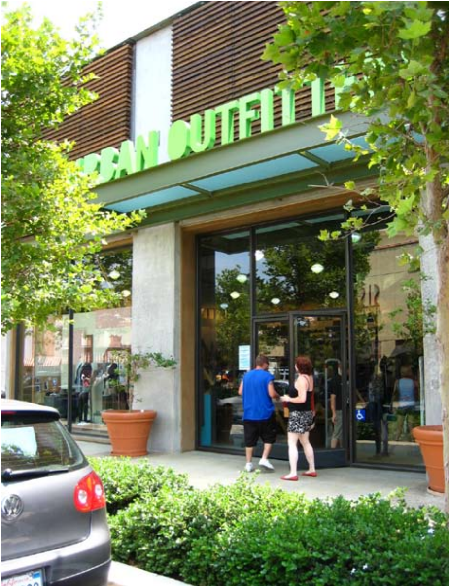
Simple detailing and envelope flashing is encouraged. Avoid excessive flashing profiles and material waste.
