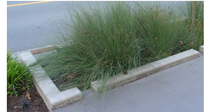
Curb inlet to collect rainwater off pedestrian path
