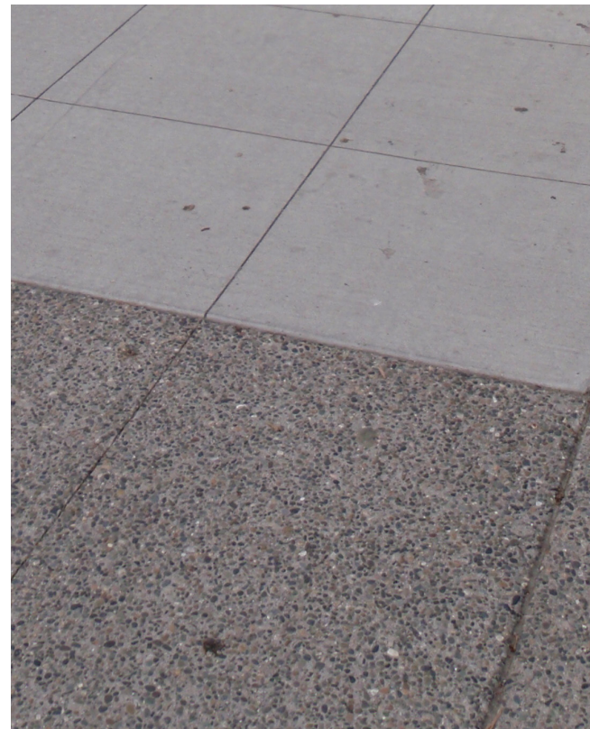
Broom Finish Concrete and Exposed Aggregate Concrete
