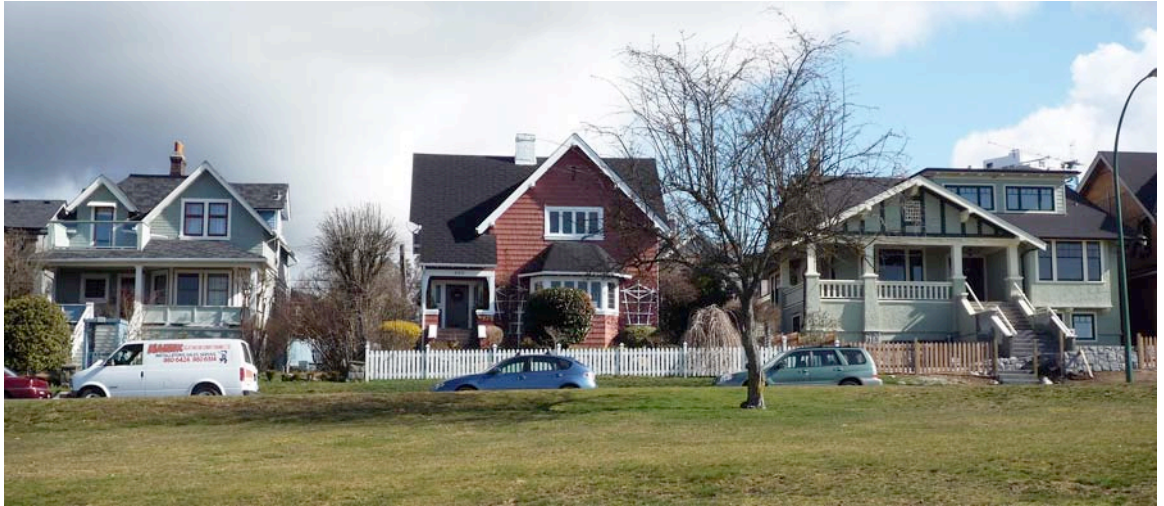
Ottawa Gardens Streetscape - North side
