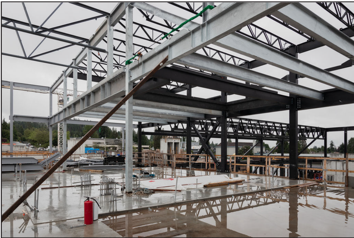
Steel construction continues (Fitness Centre)
