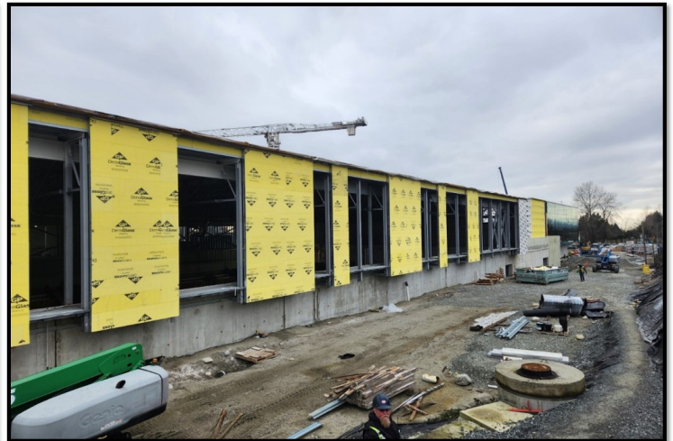
Envelope work at the Arena
