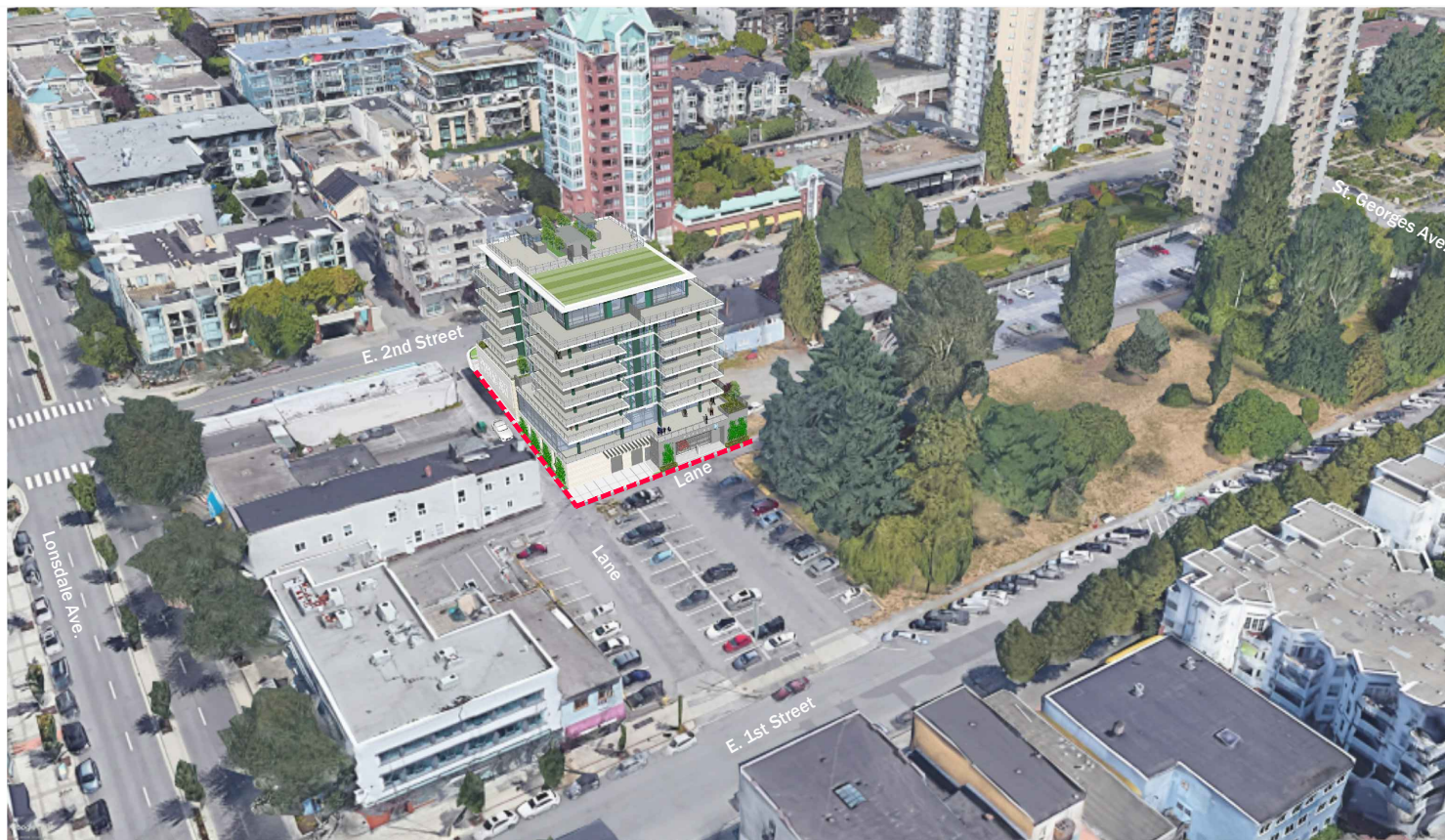
Aerial View - Southwest
