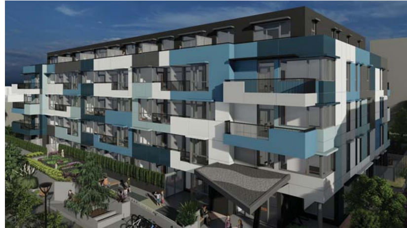
SOUTH FACADE DETAIL VIEW - SE
