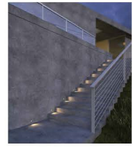
Recessed Wall / Step Light
