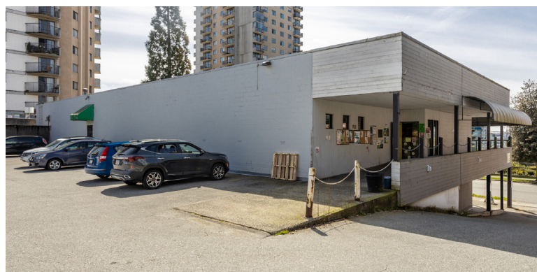
3. the back of the existing building on the site
