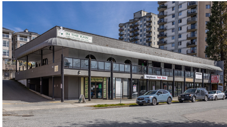
1. the street frontage of the existing building
