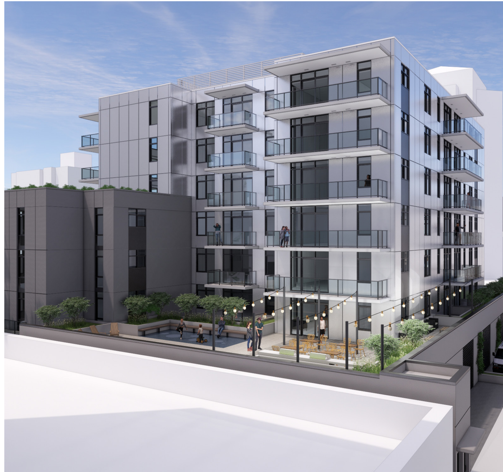
7. view of the amenity and private terraces at level 3, on top of the commercial podium
