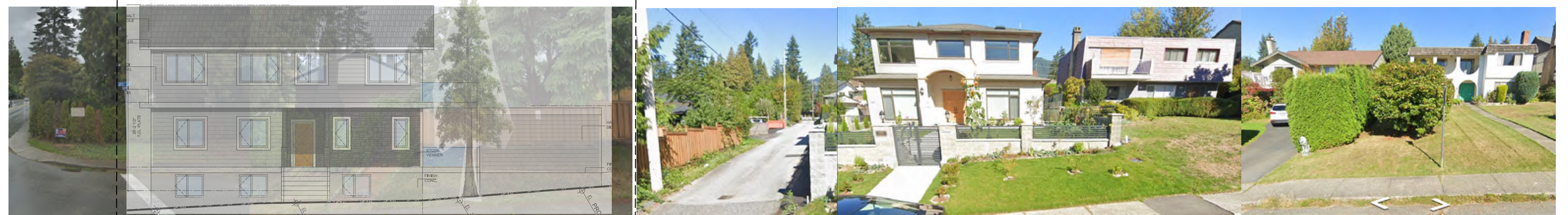
3 W 20TH STREETScape - EXISTING
