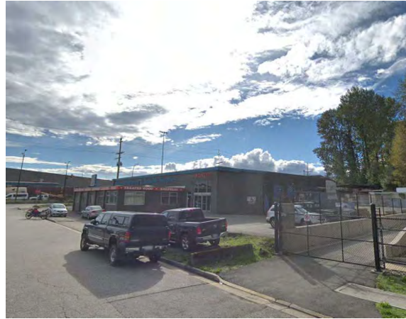
2 SITE - NORTH EAST
