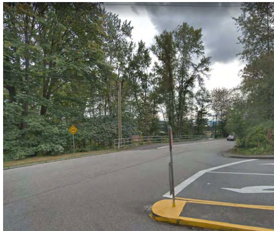
4 SITE CONTEXT - HAYWOOD STREET SOUTH-EAST TOWARDS SITE
