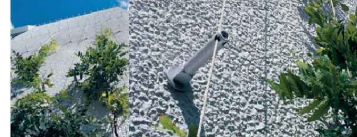
07 GREEN WALL WITH CABLE SYSTEM L9
