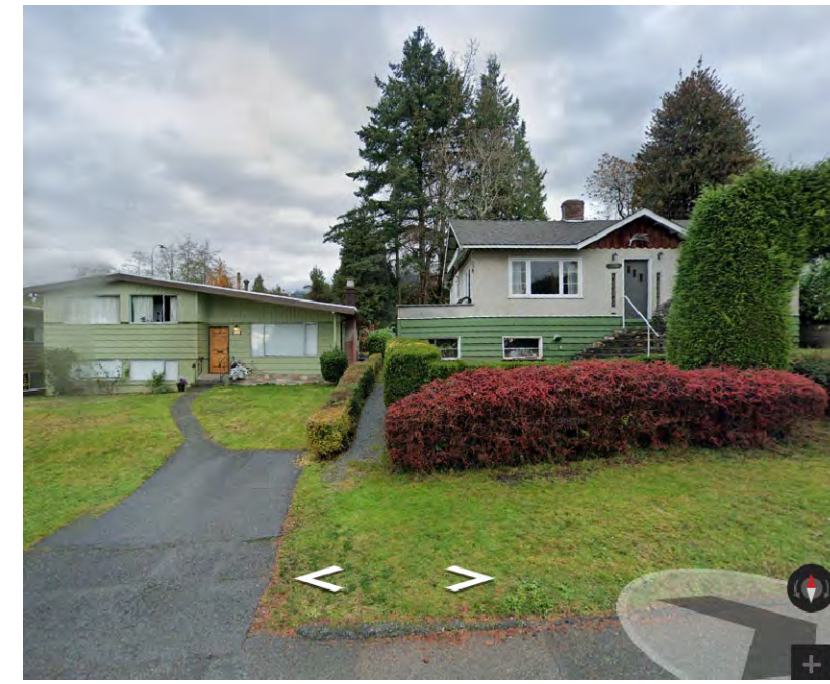
NORTH SIDE OF WEST 24th STREET
