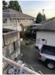
2 Retaining wall on North - View from Lane A0.13 1: 50000
