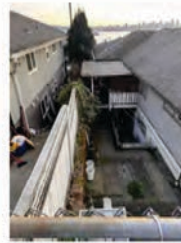
4 Existing shared retaining wall on East - middle of site A0.13 1: 150000
