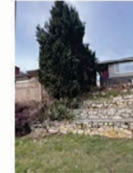
7 Existing retaining walls of adjacent site along E1st St A0.13 1: 50000
