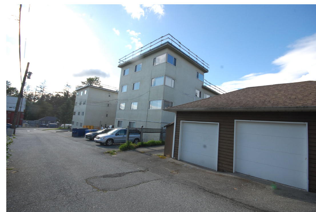
SOUTH SIDE OF LANE LOOKING WEST
