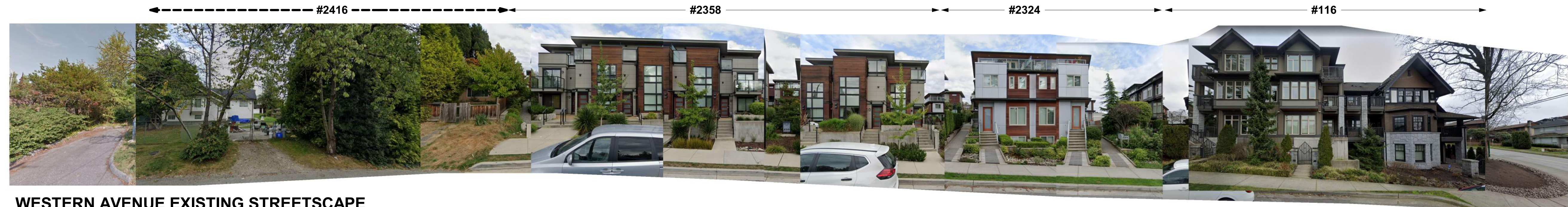
WESTERN AVENUE EXISTING STREETSCAPE
