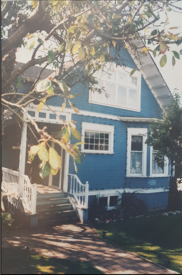
The subject house at 311 West 14 th Street in 2000. The house was painted into its current colours between 2009 and 2011. Source: MONOVA, Archives of North Vancouver, 140 [2000].
