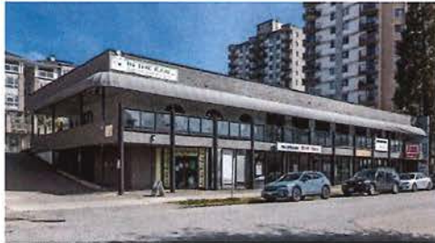
1. the street frontage of the existing building
