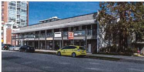
2. Eastern end of the existing building on the site
