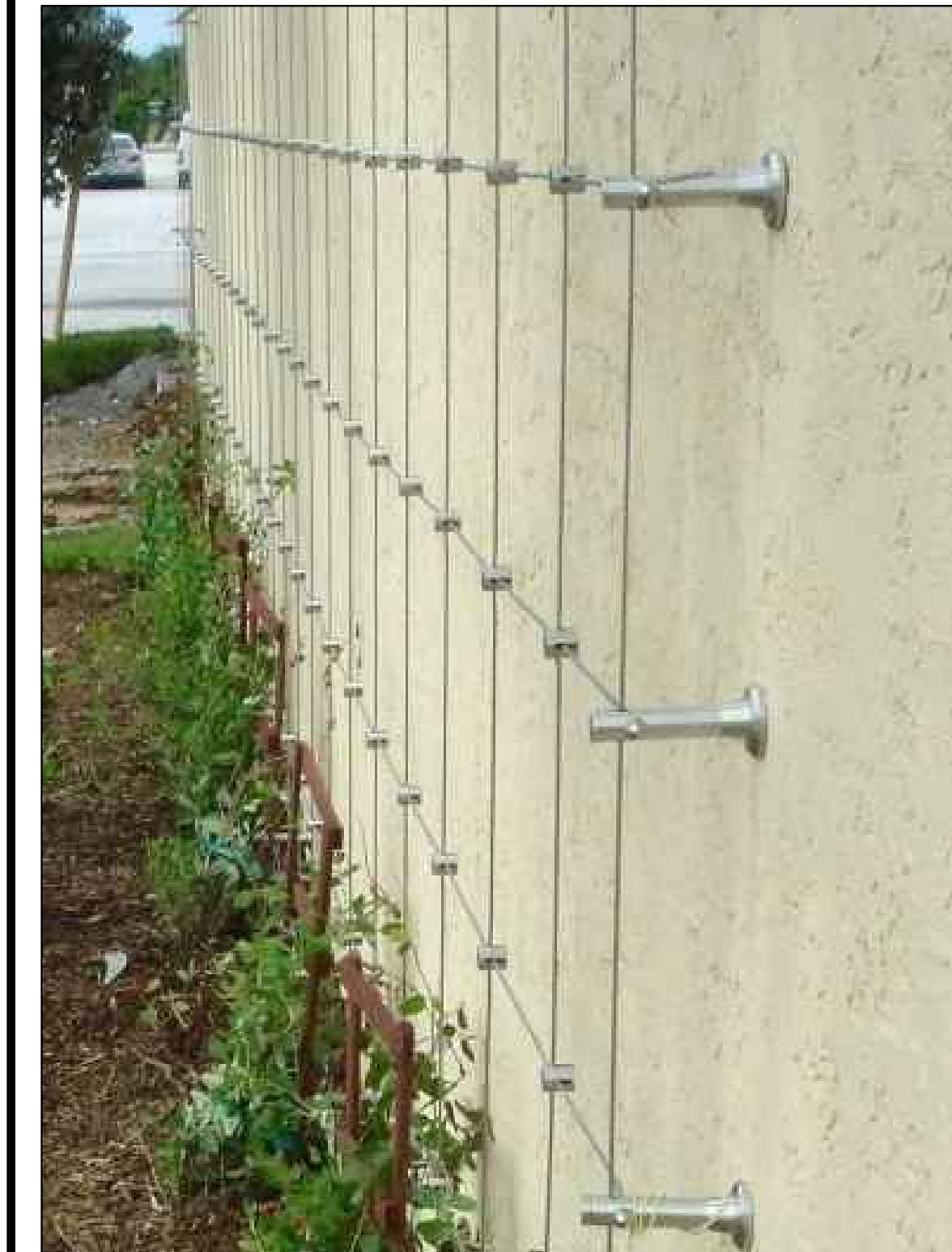
GREEN WALL CABLE SYSTEM - REFERENCE ONLY
