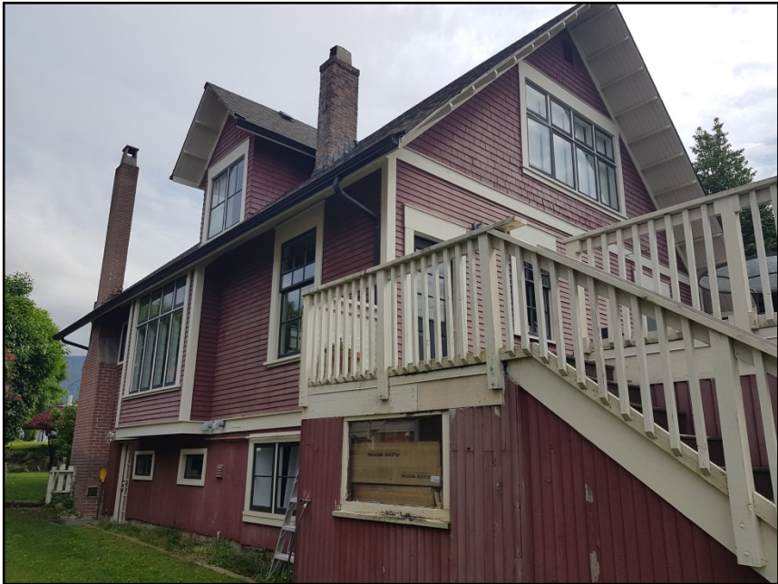
side view (west elevation)
