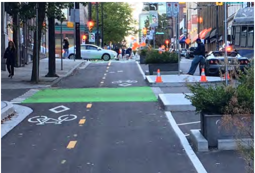
Harbourside Drive two way bike lane, asphalt, standard 2m wide bike path
