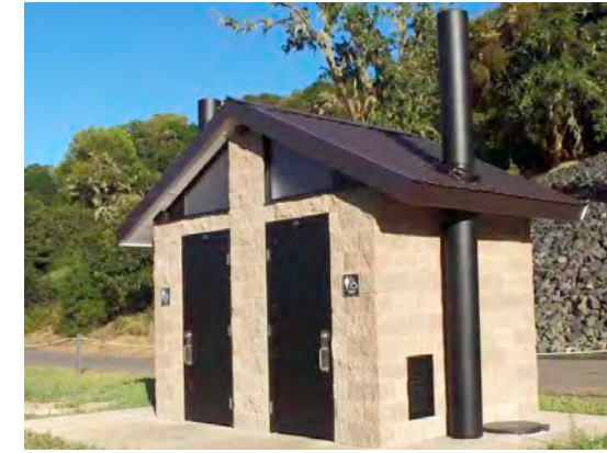
Accessible washroom facility
