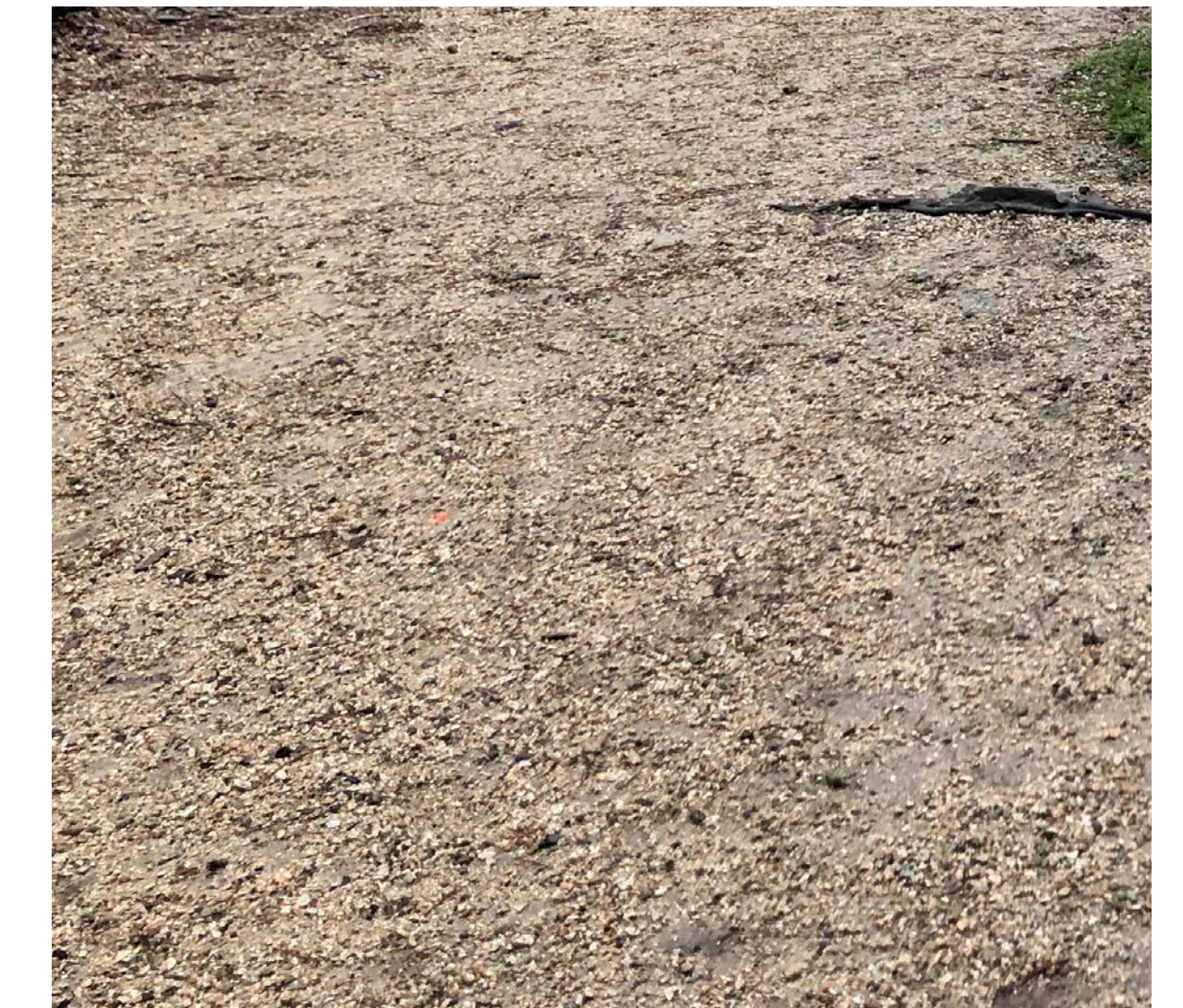
Fine crushed gravel in areas prone to high use
