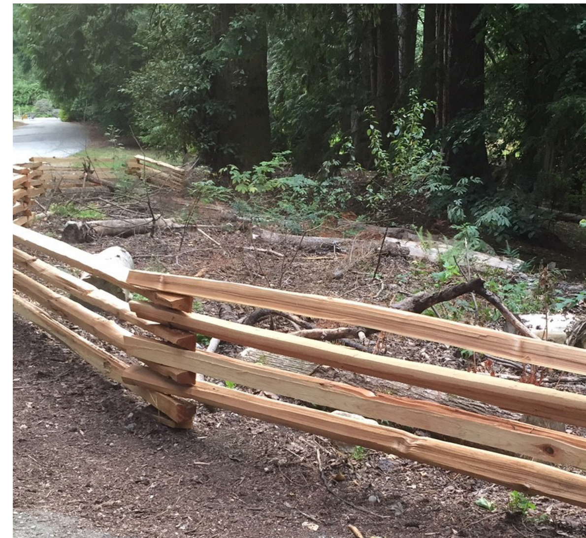
1.2 meter tall split rail fence
