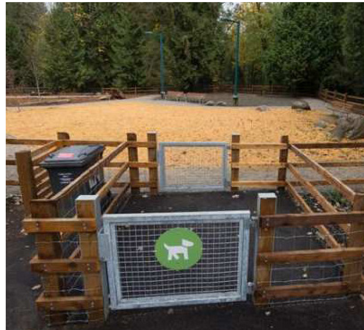
Double gate- post and rail with welded wire mesh
