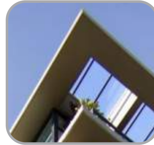
Overhanging roofs, indicating occupaiton by residents on rooftops Visual articulation of capping to mass Solar and weather protection
