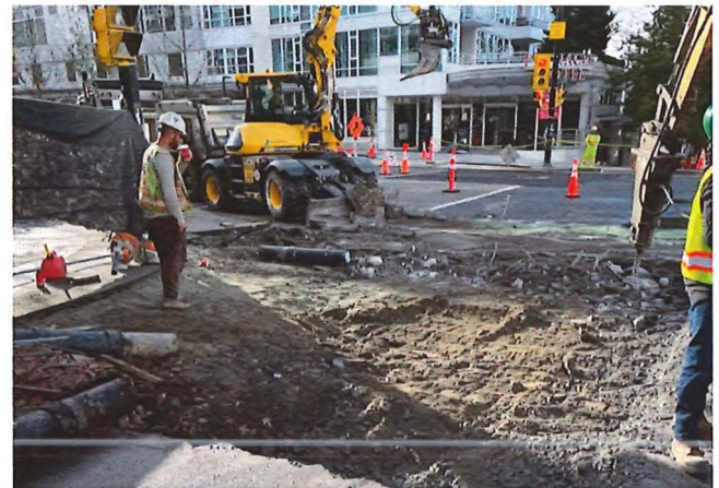
Rubber curbs and plastic delineators are replaced with concrete curbs protecting people travelling south on Chesterfield Avenue to connect to and from Esplanade on the Spirit Trail.
