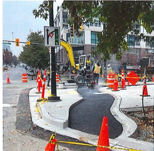
Protected intersection elements begin to take shape at Lonsdale.
