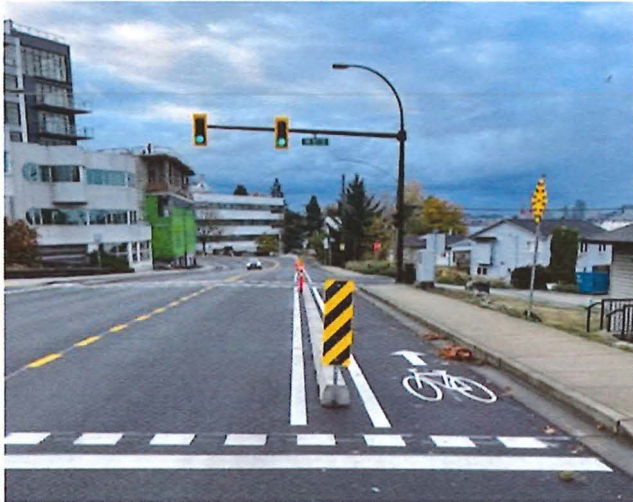
Concrete barriers now protect the southbound mobility lane on Forbes Avenue.
