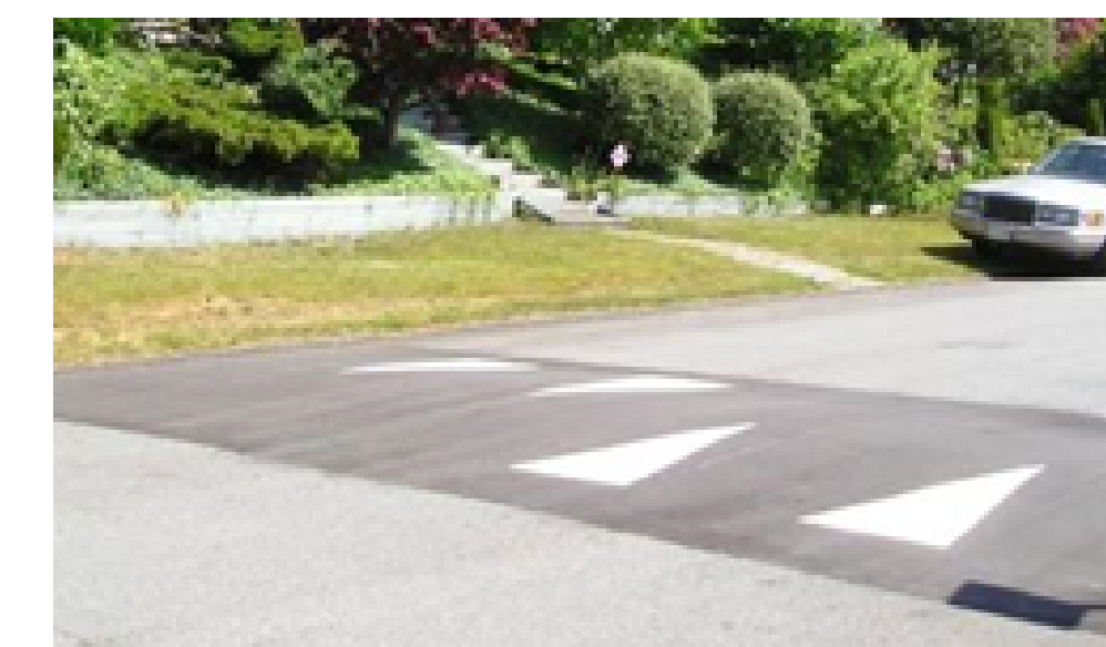
Speed humps – On a Street
