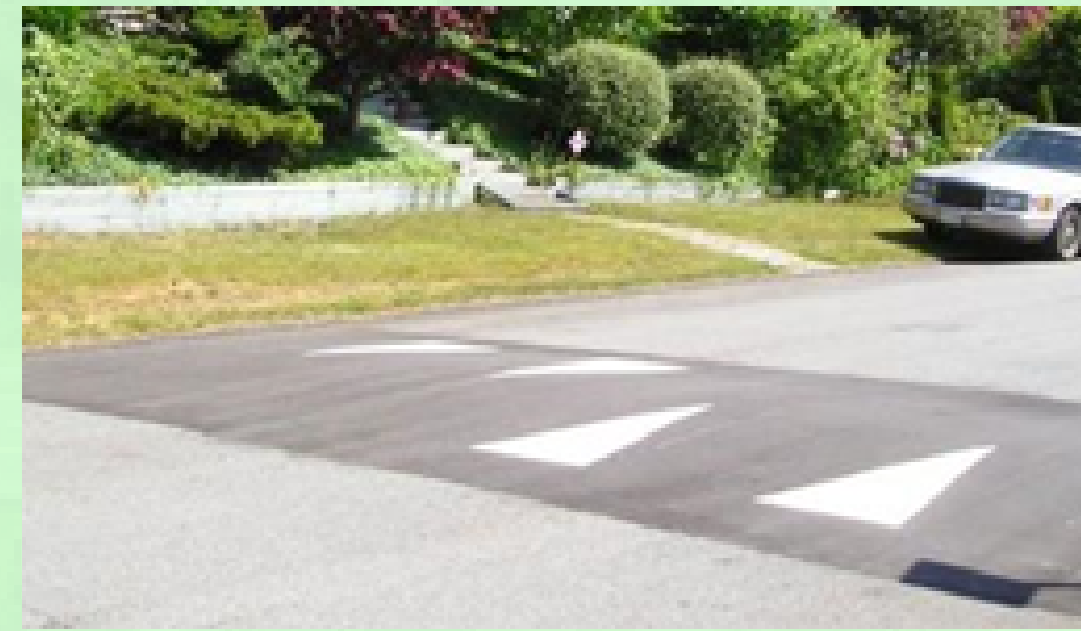
Speed humps – On a Street
