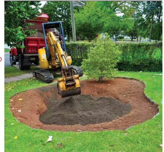
Example of residential rain garden construction (Photo: Rutgers Cooperative Extension)
