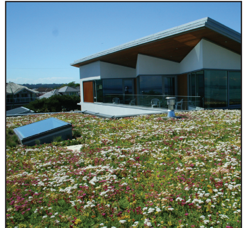
Example of green roof on Boundary Bay Beach home (Photo: NATS Nursery Ltd.)
