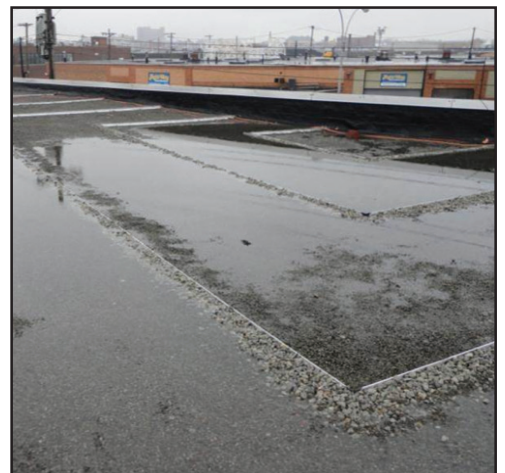
Example of blue roof in New York (Photo: Geosyntec Consultants)
