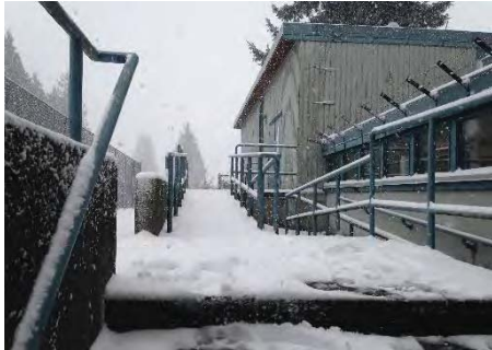
MICKEY MCDUGALL FACILITY (FIG 1)
