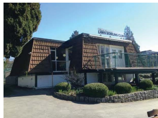
EXISTING NVLBC CLUBHOUSE (FIG 17)
